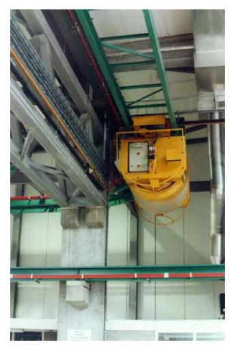
By means of the above explained kind of encoder inside the top of the conductor housing and the transmission of these pulse signals via the carbons of a collector trolley through the continuous conductor strips, the production machine and the skippers "know" exactly from each other where they are.
