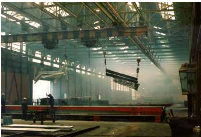
Feed and control of bridge cranes in a galvanising plant
