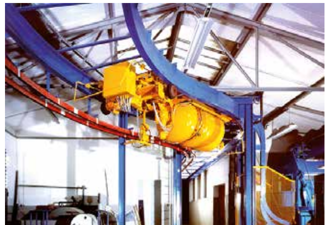
Feed and control of a concrete skipper
